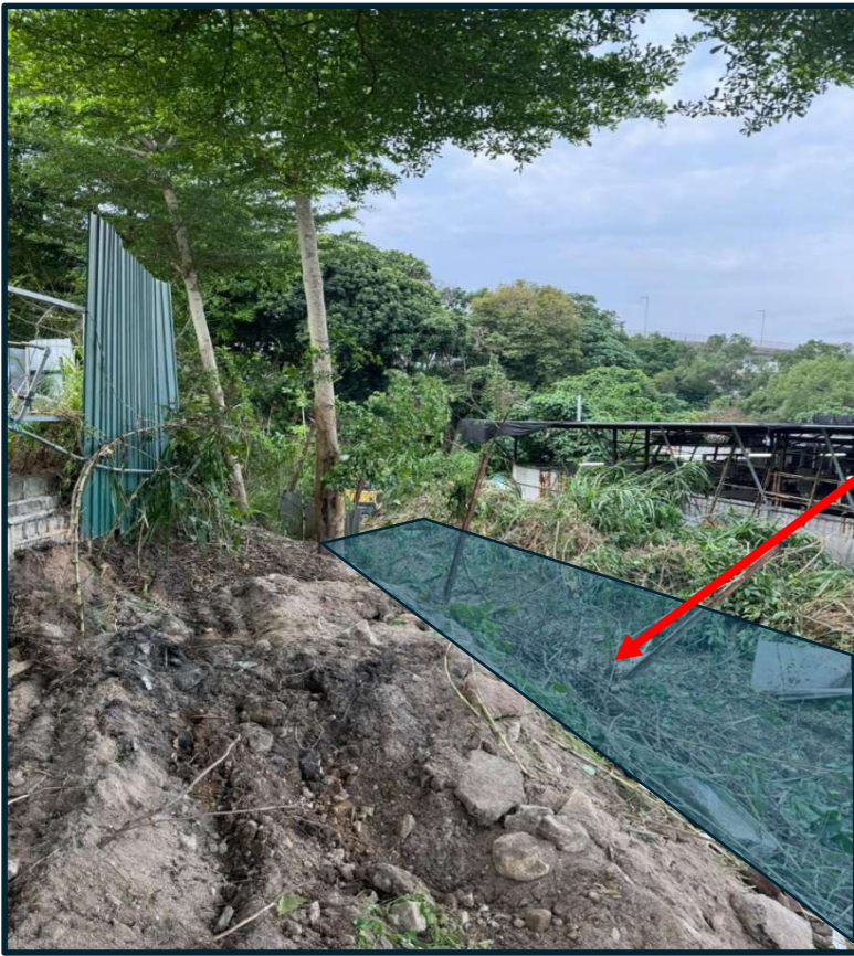
Existing Natural Stream (Dry weather), the depth is about 2m.
